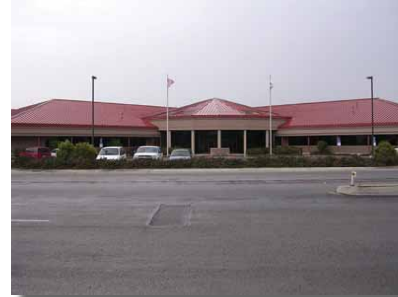
266 - Tulare Ag Building 4437 So. Laspina, Tulare, Ca
