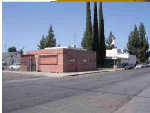
#540 - Porterville Sheriff's Substation Annex
