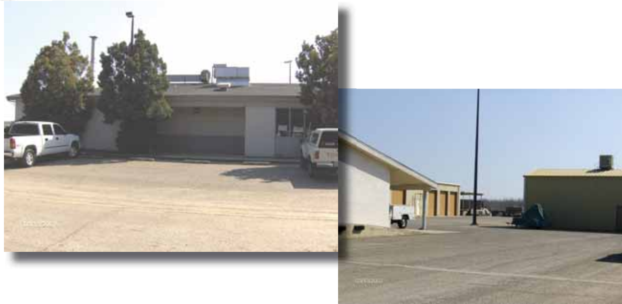
289 - Visalia Ag Warehouse 14173 Ave. 256, Visalia, Ca.
