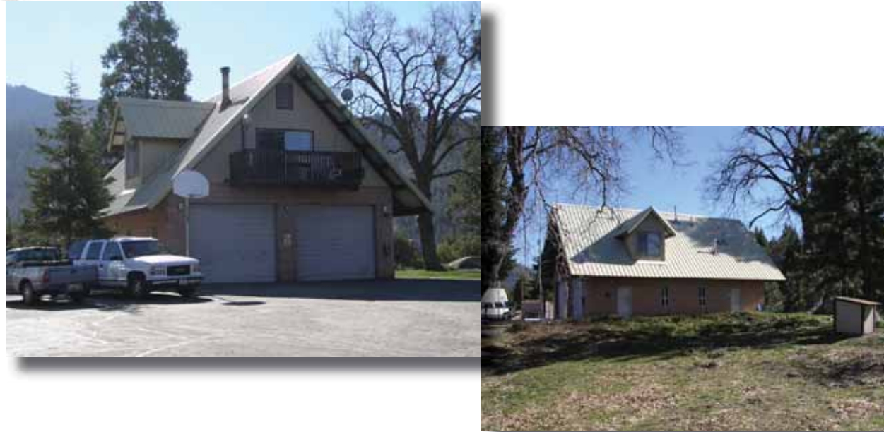
239 - Poso Fire Station 45656 Old Stage Drive, Posey, Ca.
