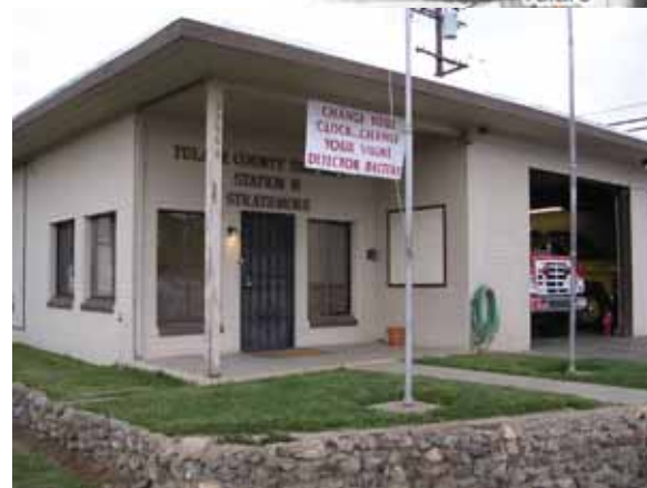
#148 - Strathmore Fire Station
